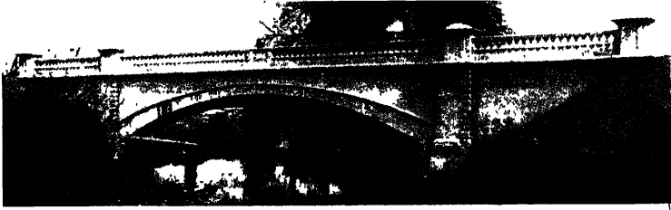
Fig. 357. Deepdene Bridge, Dorking.
